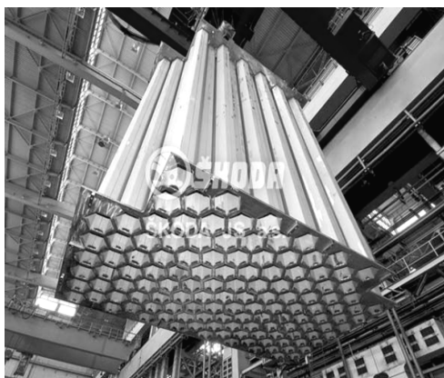
Fig. 1. Fastened racks construction to place HRP in the SFP at the nuclear power plant with VVER-1200.
