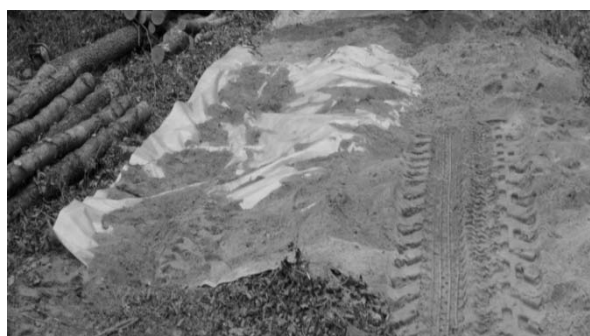
Fig. 5. Experimental road segment with geosynthetic material and brush layer
