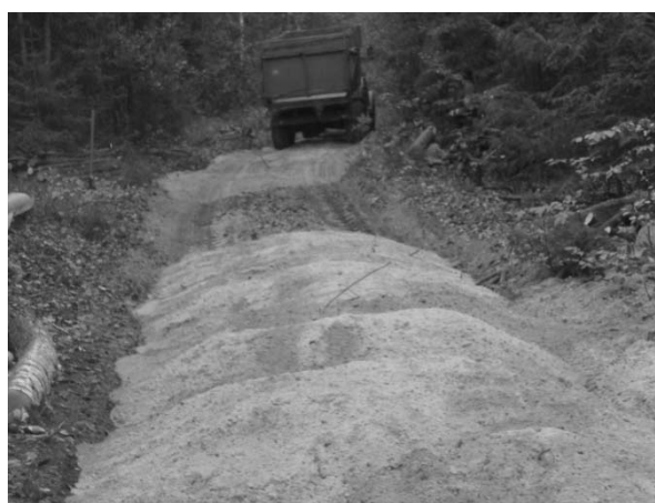
Fig. 4. Soil transportation and dumping
