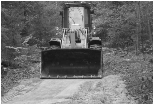
Fig. 7. Amkodor loader used to level the surface
