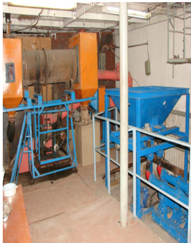
Figure 6: General view of the pilot plant.
