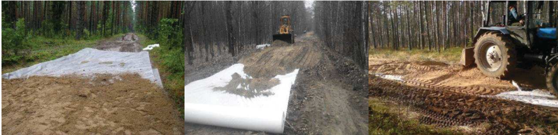
Figure 4. Construction of experimental plots with a geosynthetic layer and local soil.
