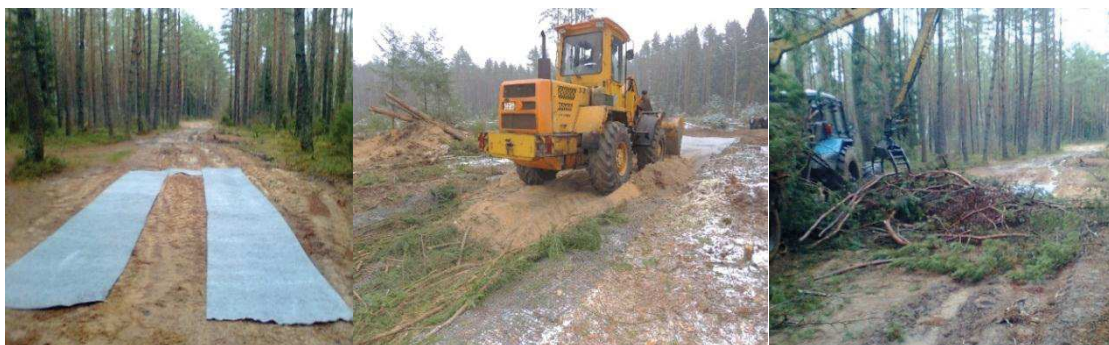
Figure 5. Longitudinal tapes and wood harvesting residues.
